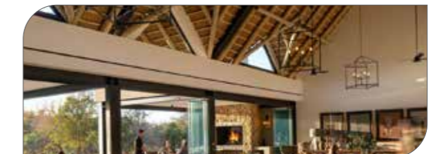
Linear slot diffusers – black linear slot on the wall above the doors.
