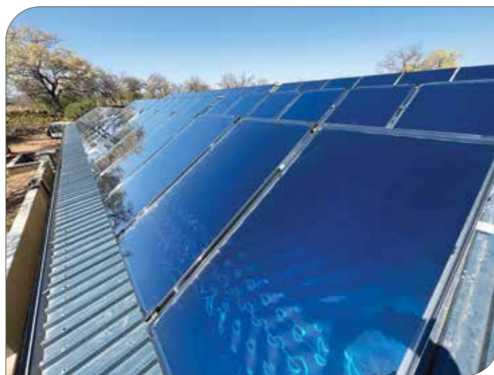
Sungazer solar hot water flat plate collectors
