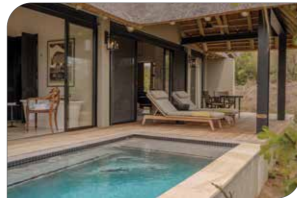
Villa pools are heated through heat exchangers.
